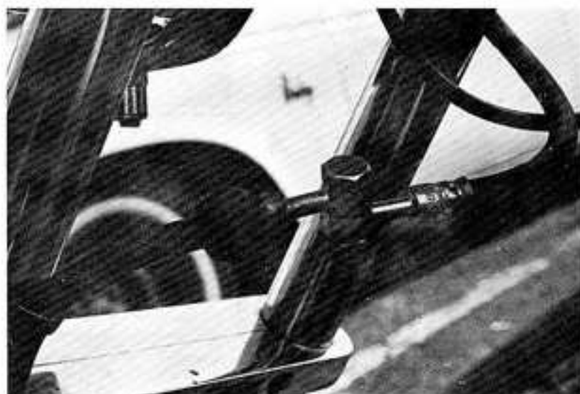
In a pinch, two hydraulic lines can be joined at the banjo fittings by a bolt but this method usually leaks.
